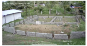
Progress on Dormitory
